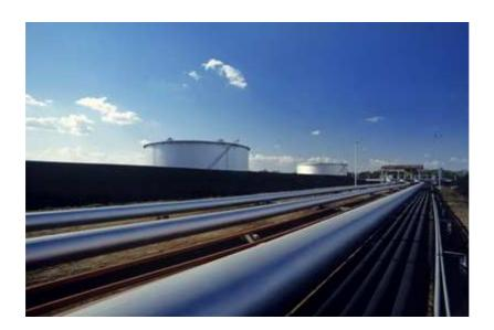
Typical applications can include pipe freeze protection, pipe temperature maintenance or heat up / start-up heating for long pipelines in tank farms, loading and unloading stations, offshore to onshore pipelines, and transfers stations.
